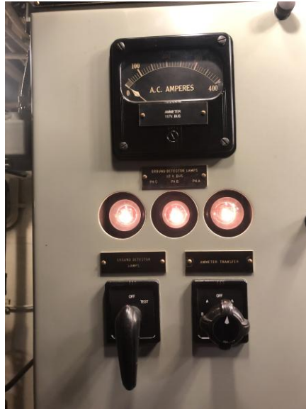
Figure 2: USS Slater (DE-766) Ground Detection Lamps (Photo by Norbert Doerry: CC BY 4.0)
